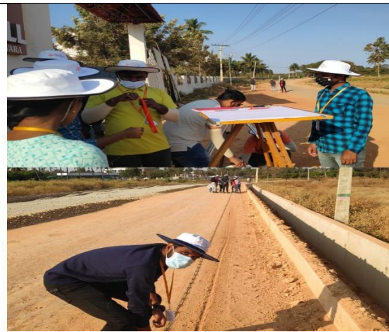
Water Supply & Sanitary work
